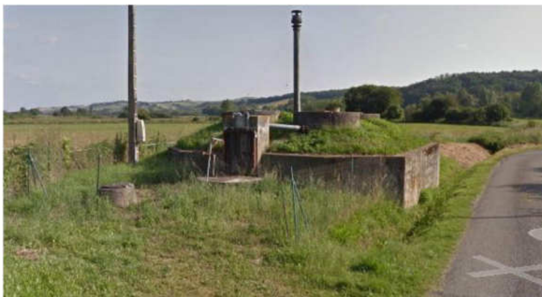
La station d'Artigat
